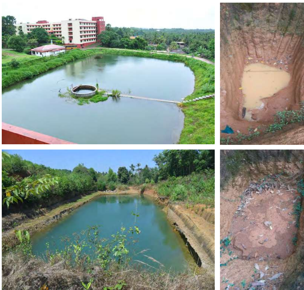
Fig 33: Rain water harvesting pond and percolation trenches
