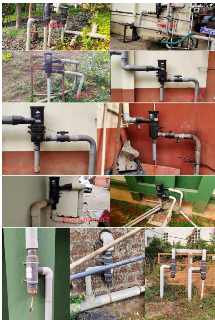
Fig 34: Roof rainwater harvesting units
